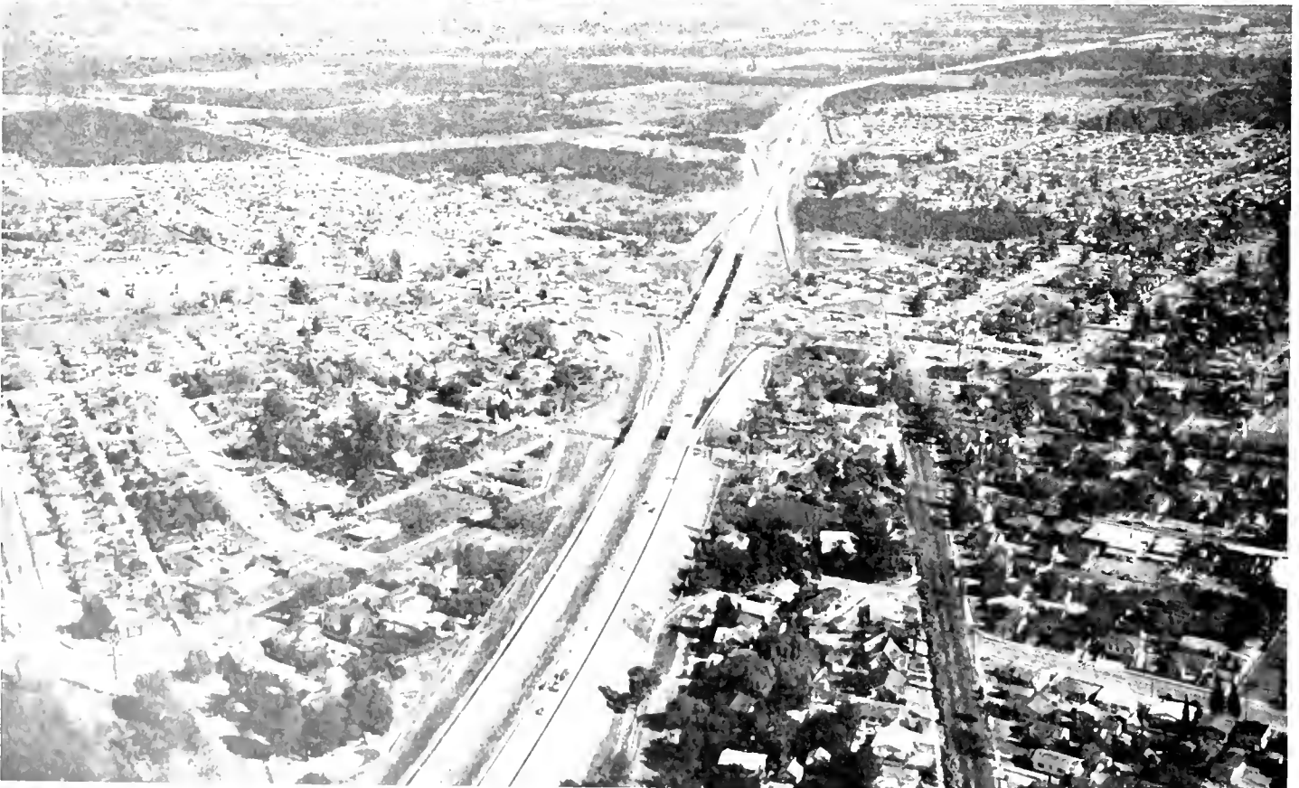
UPPER: Looking south, showing portion of San Bernardino Freeway with combination grade separation structure spanning over Garey Ave., State Sign Route 71, McFarley Ave. and Orange Grove Ave. LOWER: Looking easterly from above Los Angeles along San Bernardino Freeway with construction activities shown in foreground of Oliver Bros. Construction Company for widening bridge over Los Angeles River and Charles MacClasky for traffic interchange structure to take west-bound motorists from San Bernardino Freeway southbound on Santa Ana Freeway.
